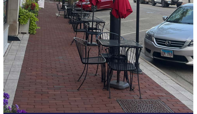
UNIT PAVERS Clay Brick Unit Paver Field: Whitacre Greer, Mulberry (15%), Dark Antique (25%), Antique (30%), Red Sunset (30%), 4"x8" Precast Concrete Paver Band: Wausau Tile, Stoney Creek, 8"x8" and 8"x12"
