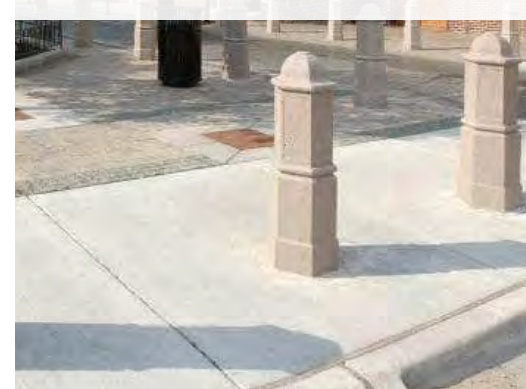
Bollard D - Precast Concrete
