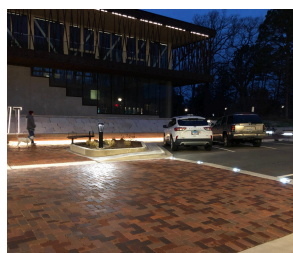
2 Integrated pavement lighting
