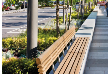
2 Bench mounted to concrete planter wall
